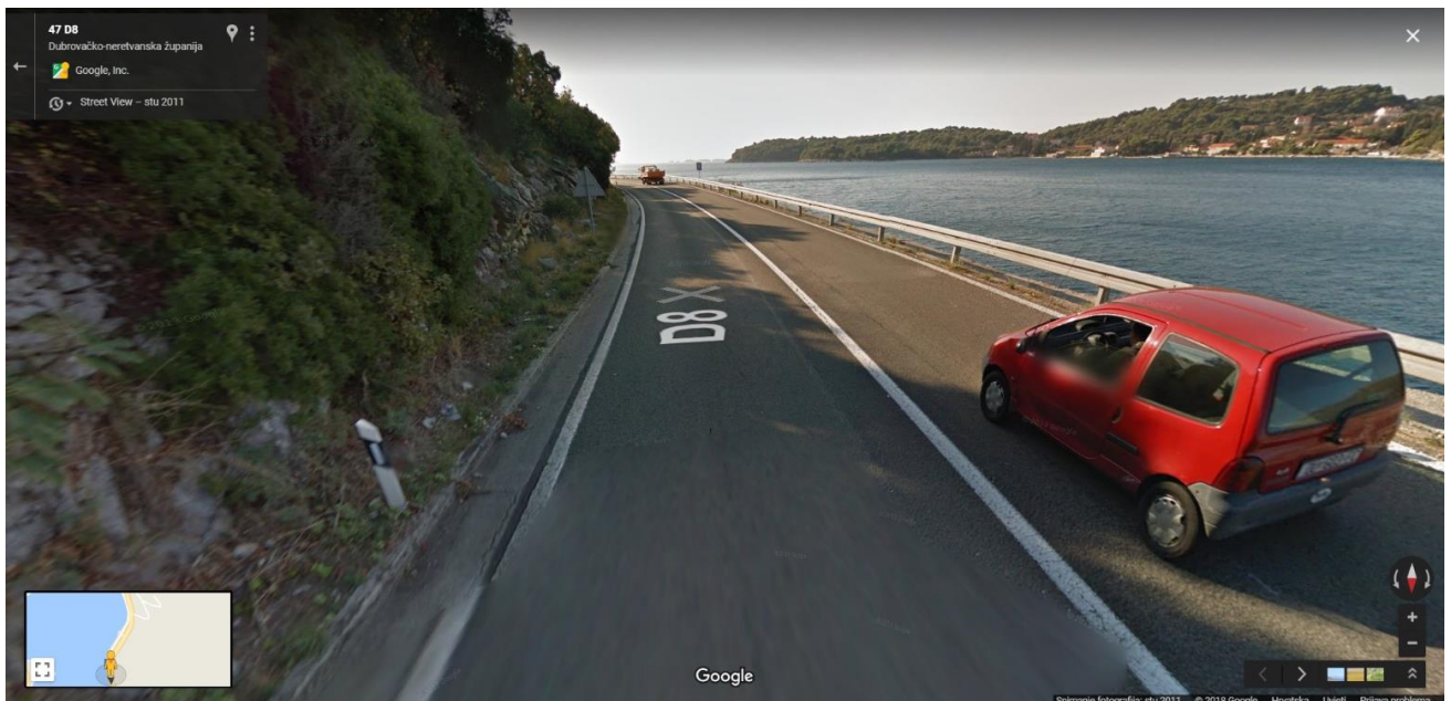
Section from Zaton to Dubrovnik bridge with high traffic
