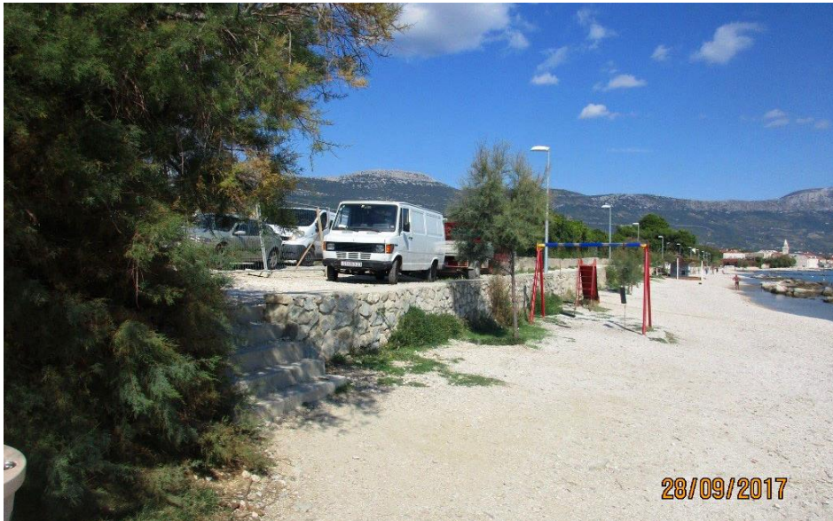
Kaštela: 5 stairs to access the road
