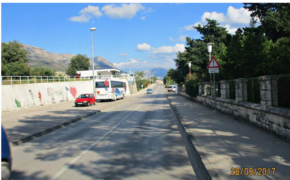
Kaštel Gomilica: road with high traffic and two wide sidewalks
